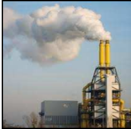
Figure I.6. Station de l'incinération [8].
