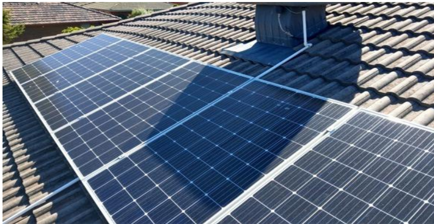
Figure.1.14 Permanent Shading in PV Systems [32]
