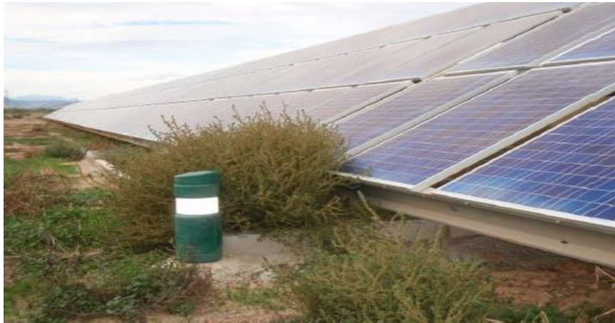
Figure.1.13 Vegetation Induced Partial Shading on PV Modules [12]
