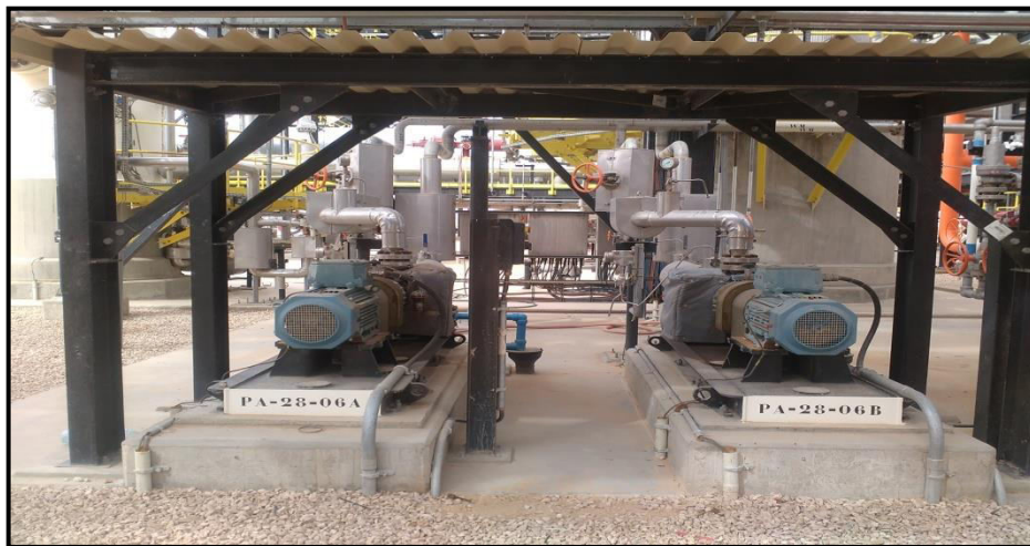
Figure II.6: Pompes booster d'amine
