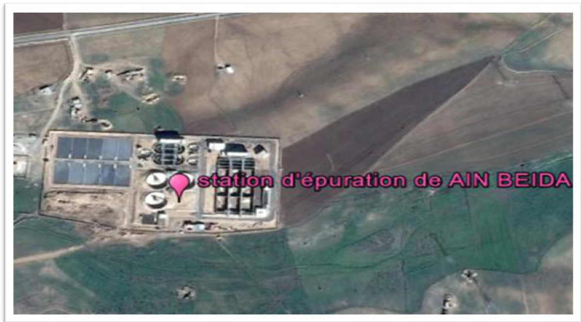
Figure 03 : Image satellite de la station de AIN BEIDA. (Google Earth, 2016)
