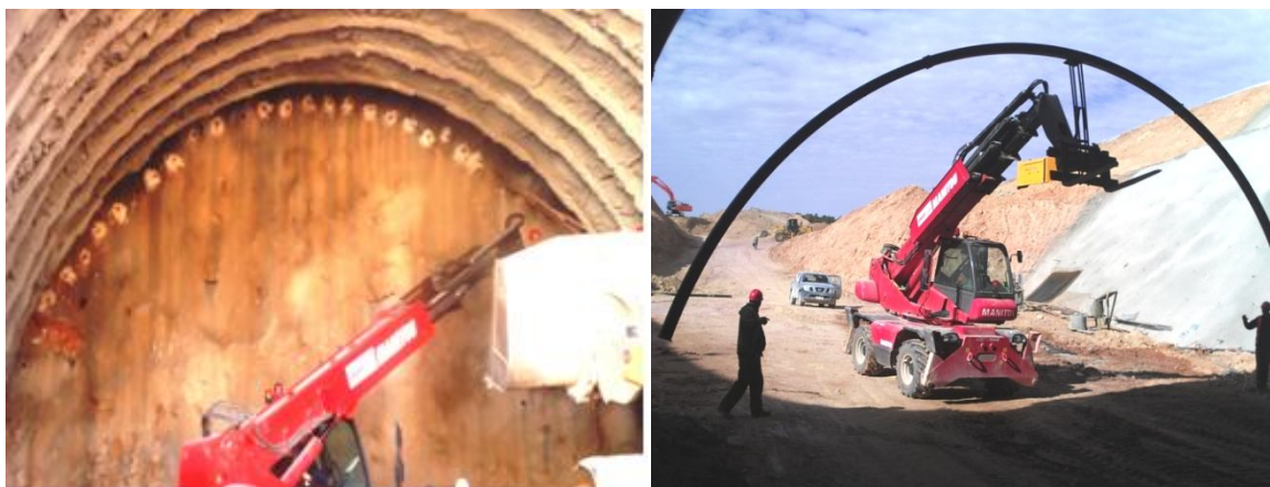
Figure IV.12: Enfilage métallique. Figure IV.13: Blindage
