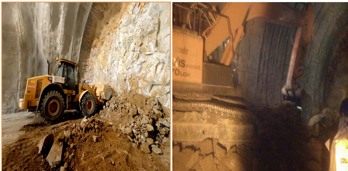
Figure III.1: photos de creusement
