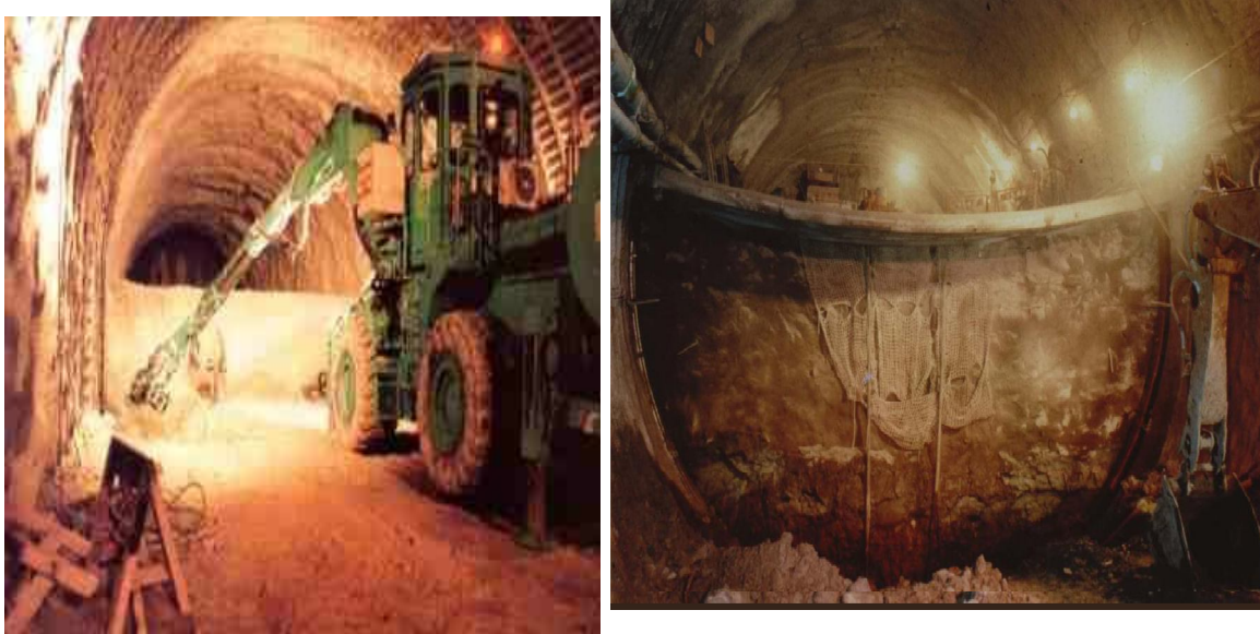
Figure III.4: creusement en demi-section.
