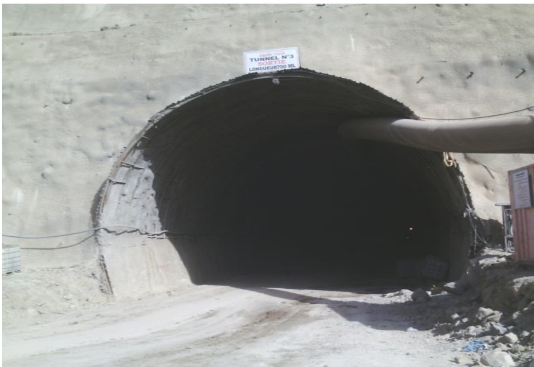
Figure II.1: photo de tunnel 3
