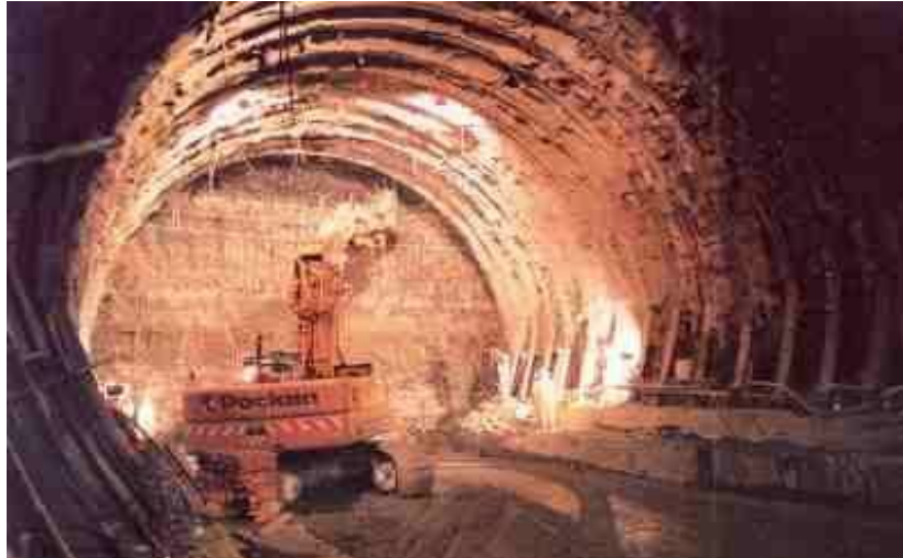
Figure III.3: creusement a pleine section.
