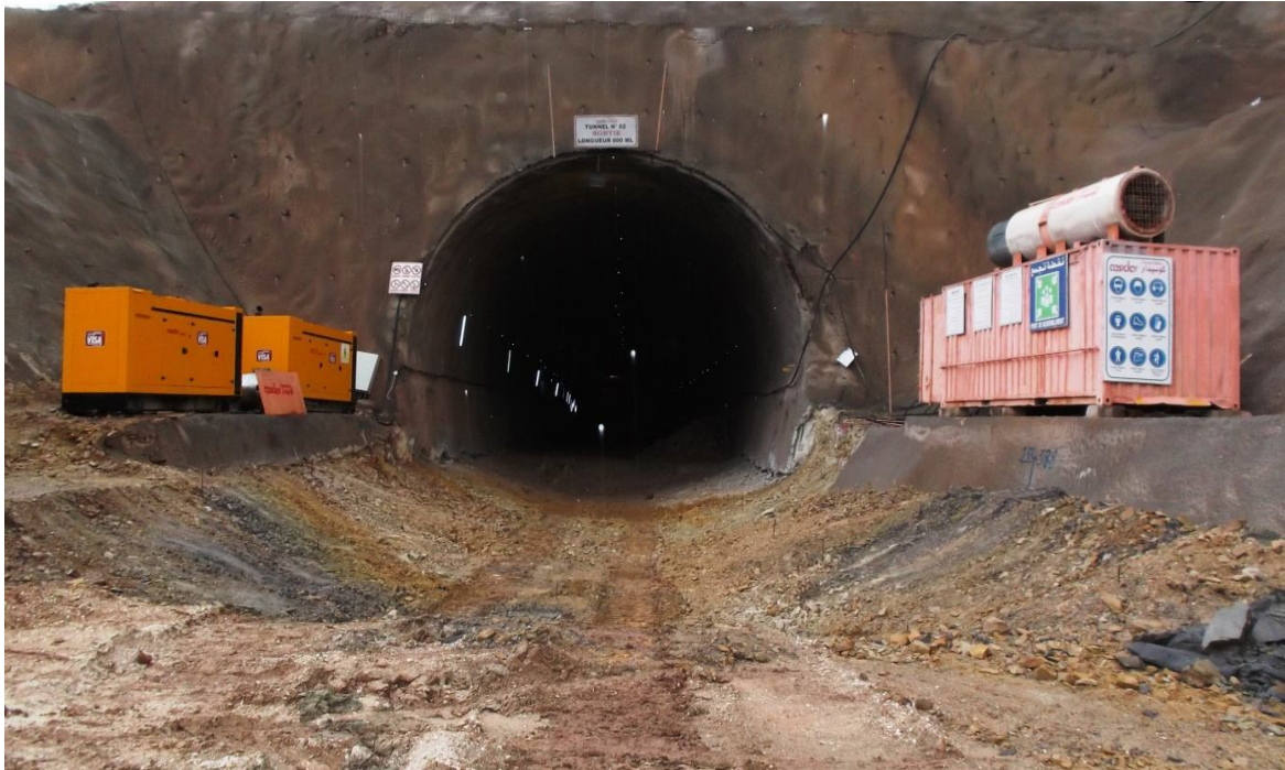
Figure I.2: photo du tunnel.
