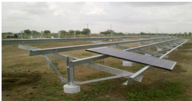
Fig.II. 6. Example of block type foundation
