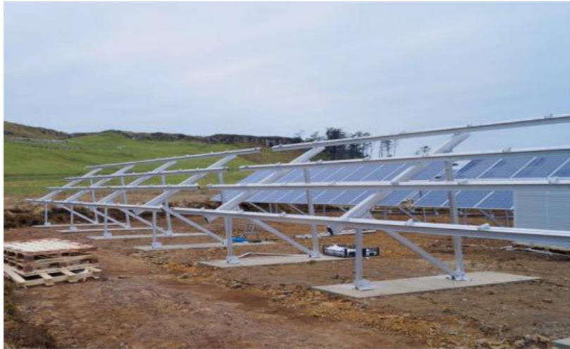
Fig.II. 7. Example of slab foundation
