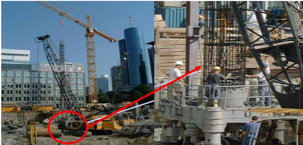
Figure II. 5. Assembly of reinforcement cage [94].
