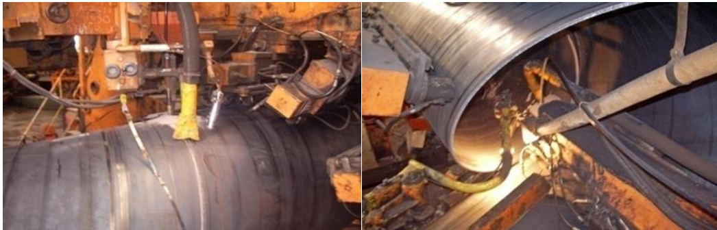
Figure 1.9: Tube Welding(M. Nahal, 2016)
