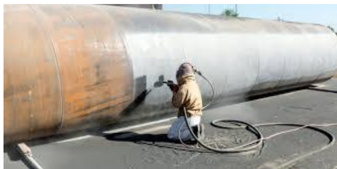
Figure 1.14: Pipeline sandblasting
