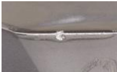
Figure II.11 : Usure mécanique (Ecaillage).
