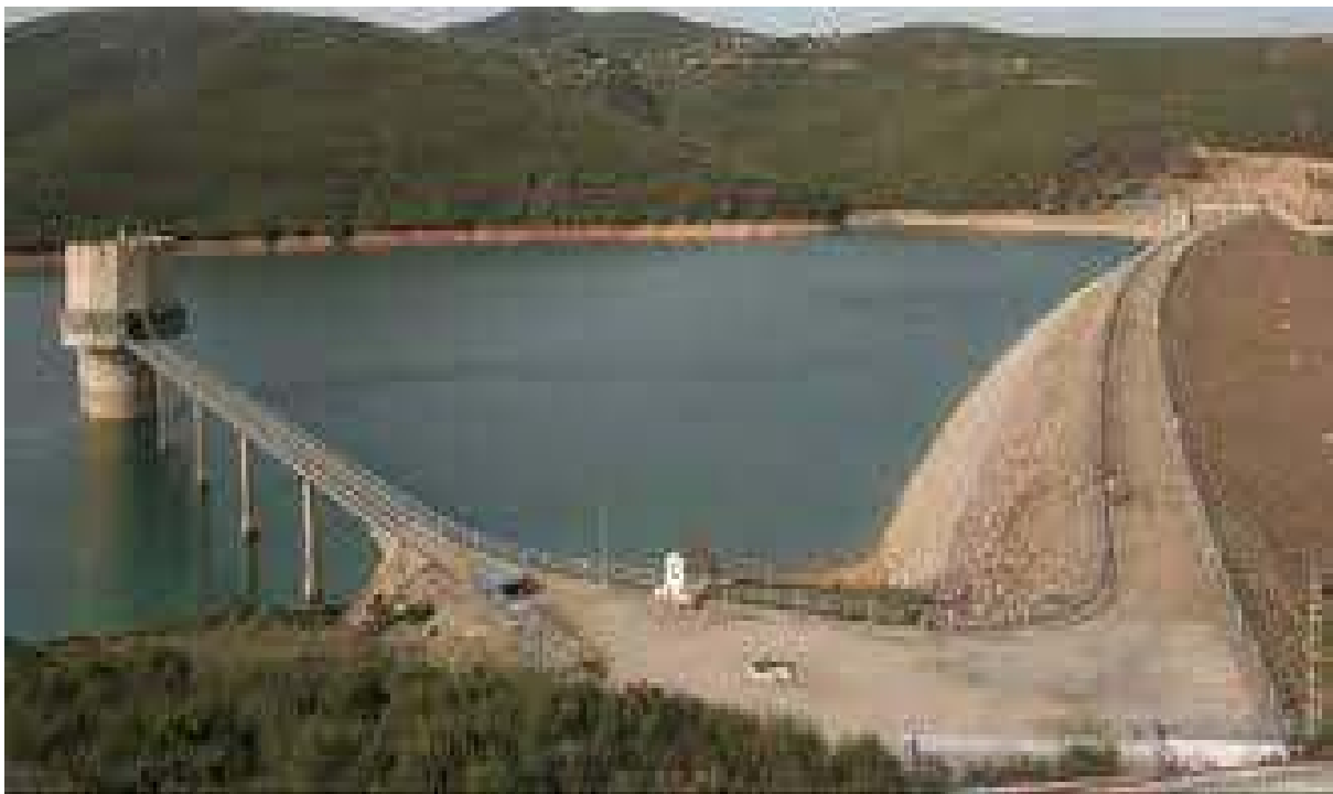
Figure 3: Le barrage d'oued charef.
