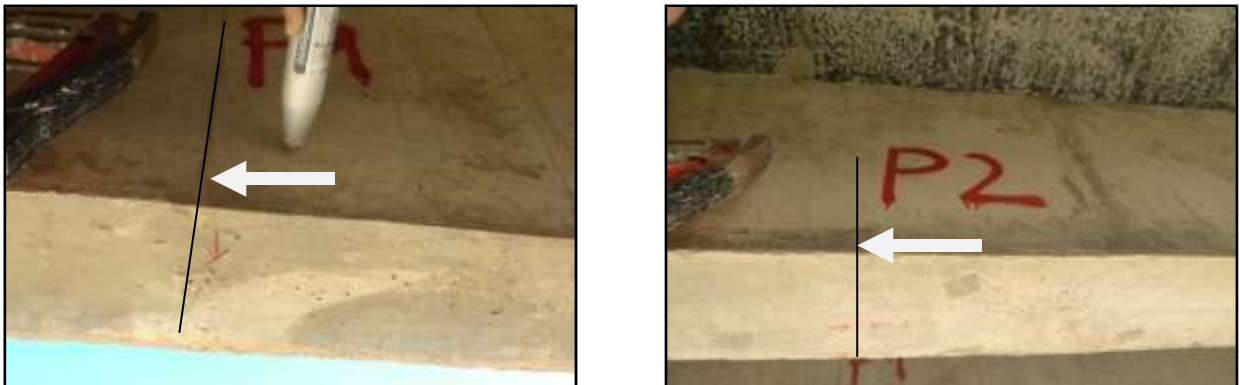
Figure 4.6 : Fissures verticales
