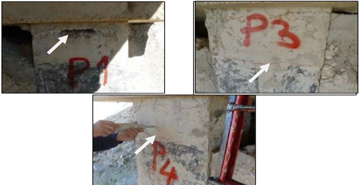
Figure 4.11 : fissures horizontales
