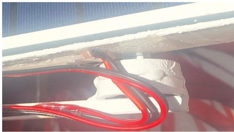
Figure 4.2 installation des LDR
