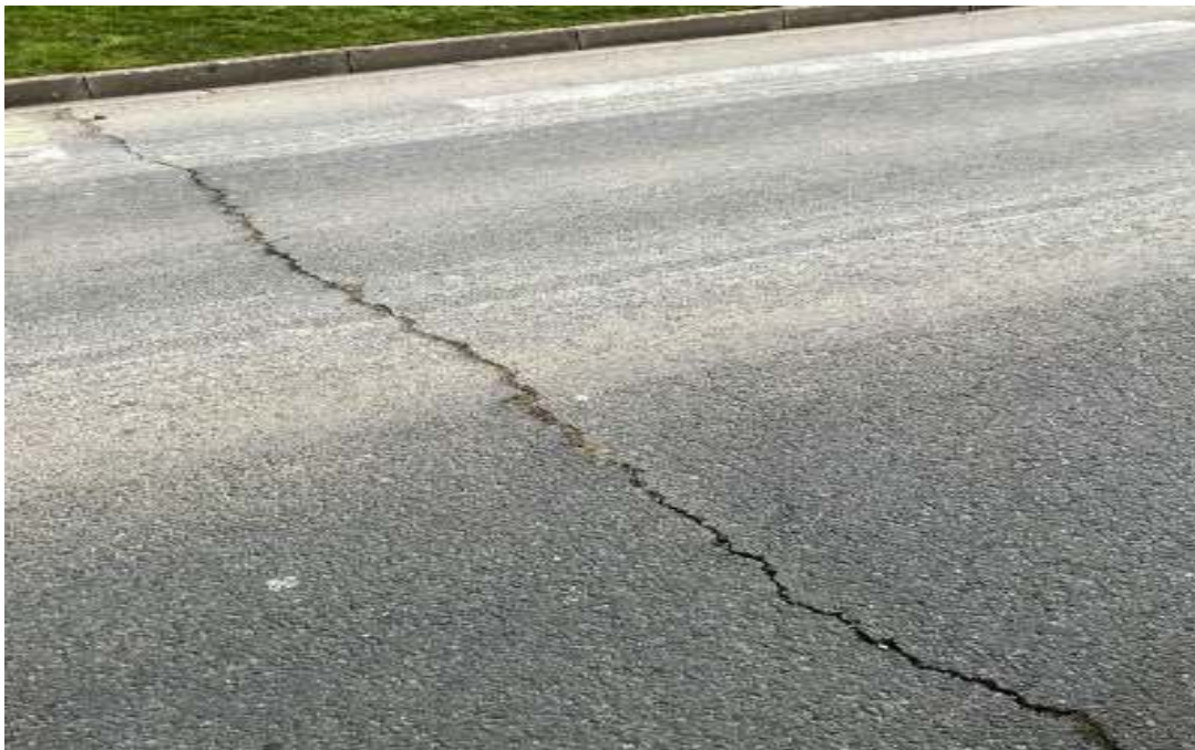
Figure XXI: Fissuration transversale
