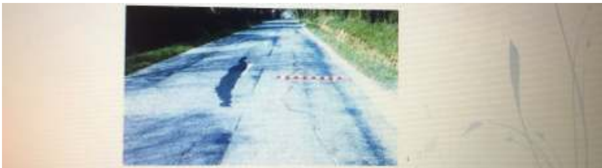
Figure XXIV: Fissuration d'adaptation
