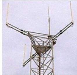
FIGURE II.4 – Antenne omnidirectionnelle.
