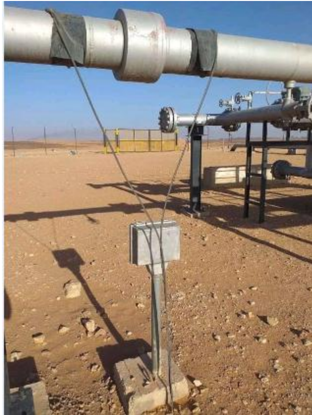
Figure III.11 : la Protection cathodique
