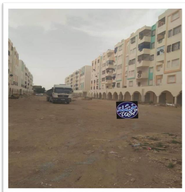
Figure (30) : Cité784 Logements
