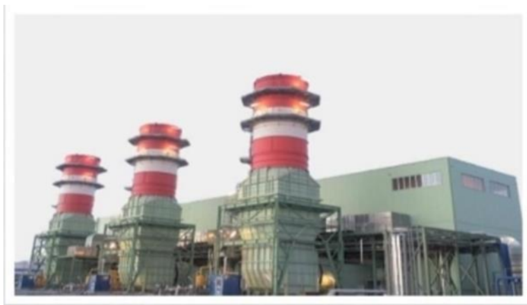
Figure 1: Centrale TG de LABREG (3x140,5 MW).
