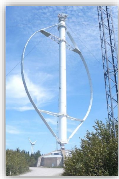
Figure 12: Darrieus Type rotor (VAWT)
