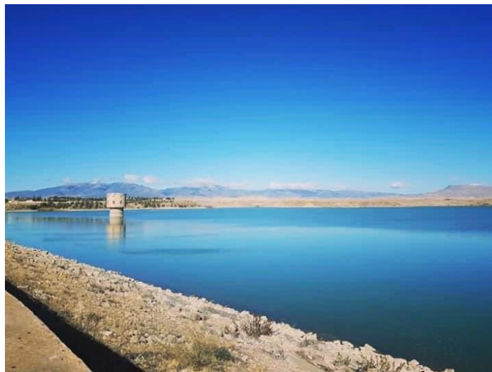
Figure III.1: Barrage de Babar
