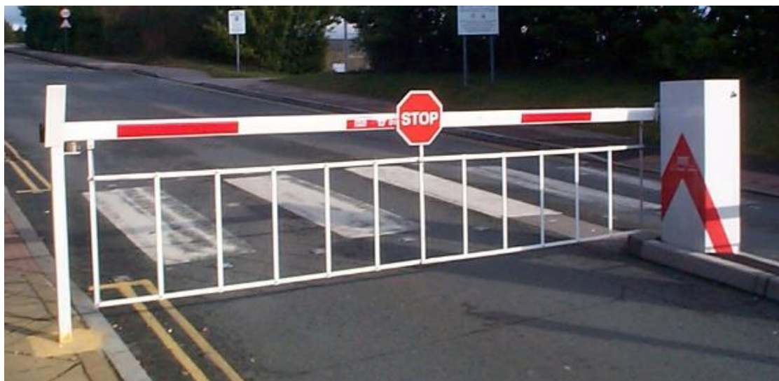
Pic 10 .....FBX rising barrier
