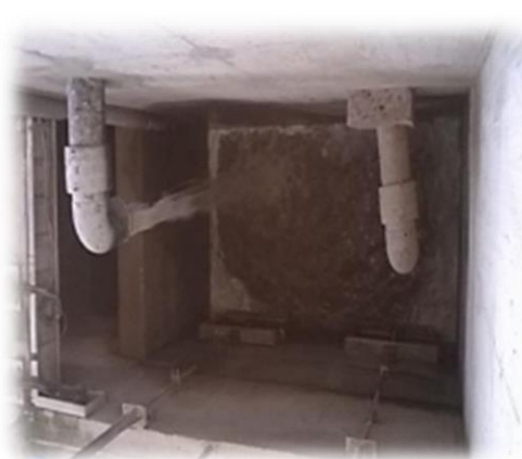
Figure III.5: Pompes de relevage
